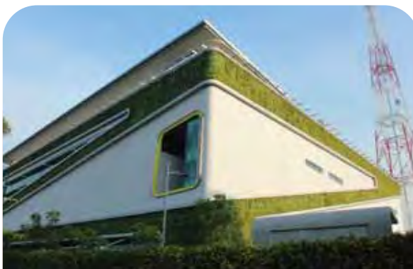
DiGi's Technical Operations Center achieved full Gold Certification from the Green Building Index (GBI). In 2012, GBI auditors verified that various eco-friendly features indicated in the planning and design stages of the building were effectively implemented.
